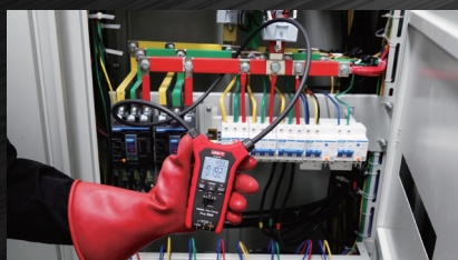
Bus bar current test
